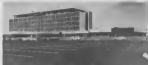
Administration, Ambulance Building, 262 beds Patient, 200 Card, and 200 General Medical Director building at the new hospital.
